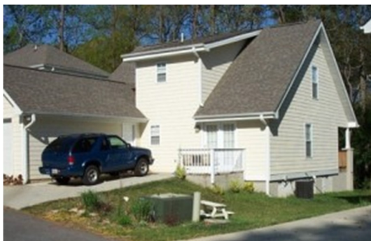
A visitable home featuring a zero-step back entrance. The zero-step entrance need not be to the front of the home and can be placed over basements.
